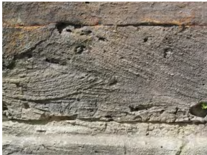
Stone at the Roman Baths, Bath: a) the base of a Roman column with a bolt-hole cut into the top; b) a block of Roman stone with cross-bedding and burrows.
